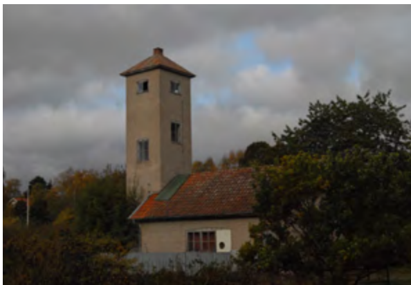
Brandstation i Halltorp
